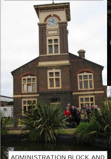
ADMINISTRATION BLOCK AND CLOCK TOWER
